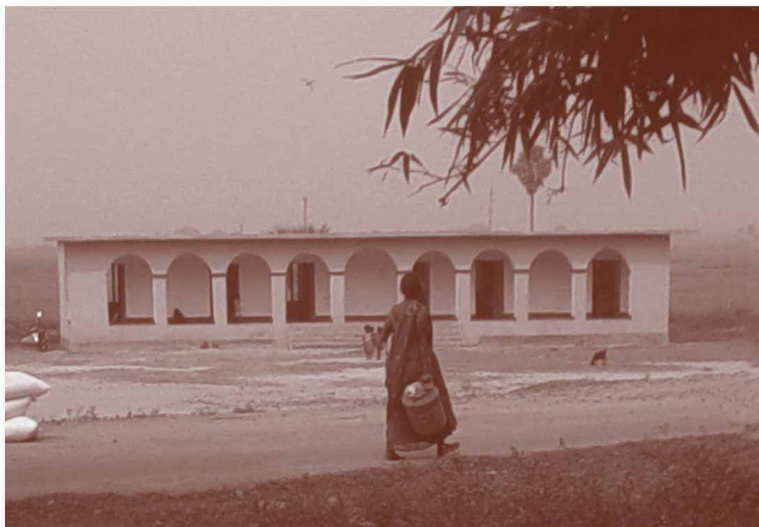
Newly constructed classrooms in Majhauri School
